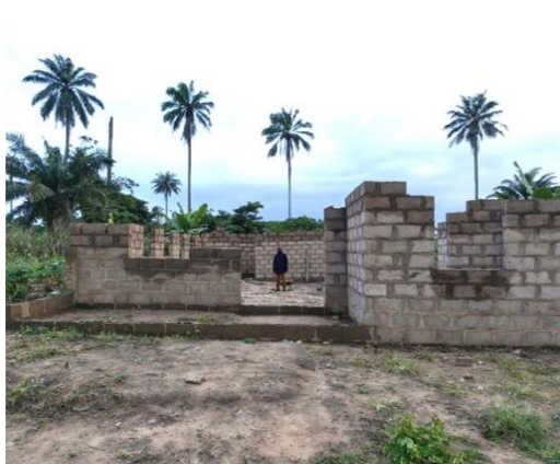
Church building in progress at Oba village. A work of faith, trusting God to complete.
